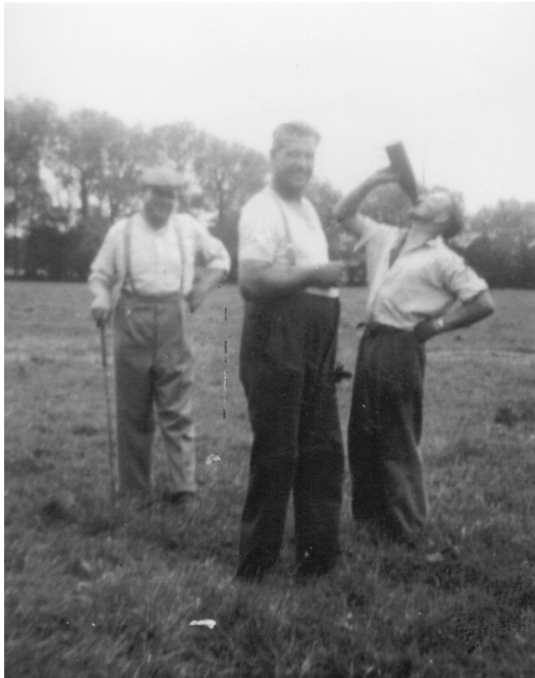
A photograph thought to have been taken when the railway equipment was first delivered to site of the railway in May 1944. Left to right: the farmer who owned or leased the land, Ernie May ("Dosher") and George Gould. Ernie and George were both employees of Harold and are enjoying some liquid refreshment. Ernie was a great steam enthusiast.
